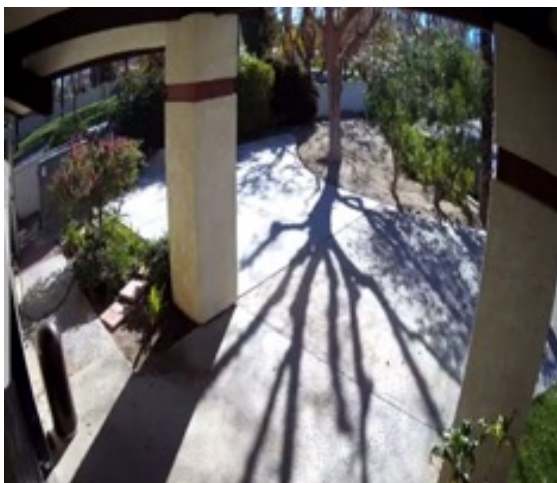
Front of Pump House
